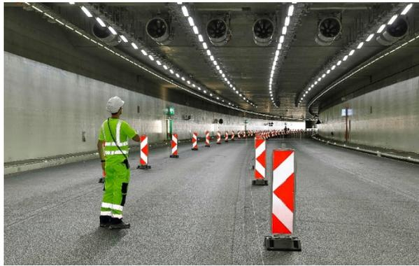
**Figure 6: Jet-fan battery in the Nord tube of the tunnel Katzensee (Source: FEDRO).**
