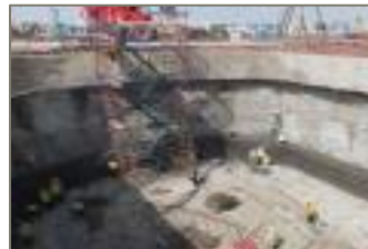
Start shaft for TBM
