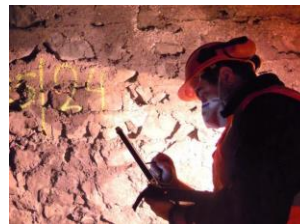
Use of a touchpad for tunnel inspection
