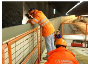
Inspection of a road tunnel
