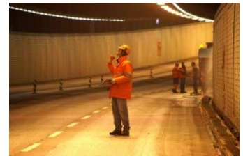
Visual inspection of the ceiling in a road tunnel
