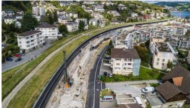
Renovation Project A2 Hergiswil
