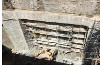
TBM starting wall
