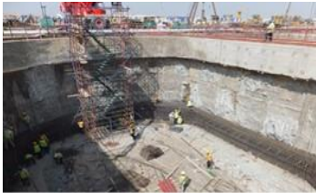
Start shaft for TBM
