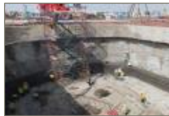
Start shaft for TBM
