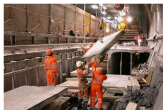
Construction works at the San Bernadino Tunnel
