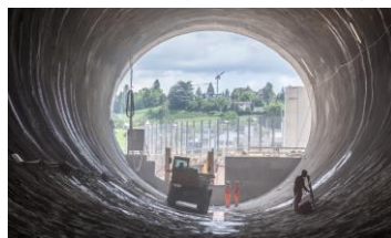
Tunnel portal Galgenbuck Tunnel
