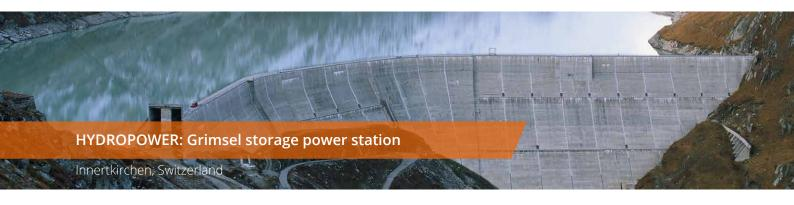
The Grimsel 3 power station is primarily used to adjust electricity production to current demand at short notice. Surplus electricity is used to pump water into higher-lying lakes. As soon as the demand for electricity increases, the power station can generate up to 660 MW of electricity again.
