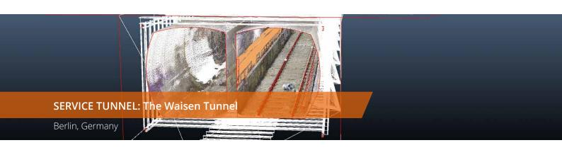
The existing Waisen Tunnel under crosses the river Spree in the centre of Berlin. It serves as an operating tunnel connecting the U5 and U8 lines. Built in 1917, it is a piece of contemporary history that needs comprehensive renovation.
