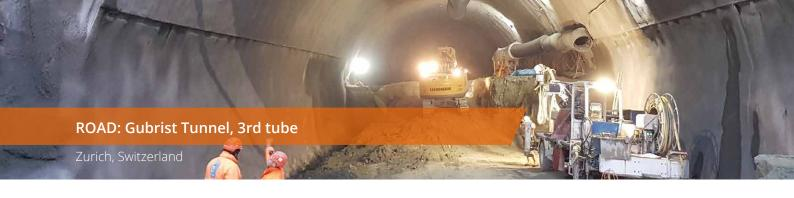
The expansion of the Zurich northern bypass is a key project in the Swiss motorway network and contributes significantly to better mobility in the Zurich area. A third tunnel tube supplements the two existing 3,250 m long road tunnels.
