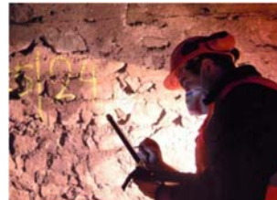
Use of a touchpad for tunnel inspection
