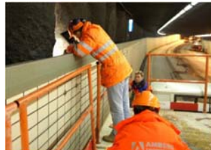
Inspection of a road tunnel
