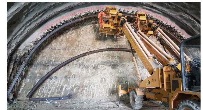
Installation pipe screen
