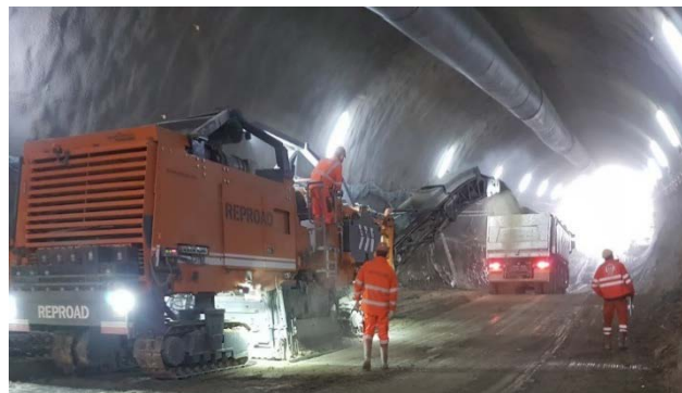
Dismantling bench using a rock cutter
