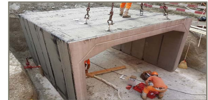
■ Service tunnel elements (WLK)
