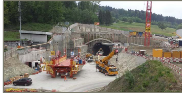
Driven portal side Affoltern
