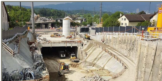
■ Execution lid construction Weitingen
