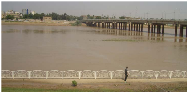
■ Bridge crossing Karoon River
