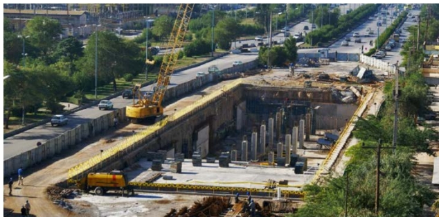
■ Start shaft for TBM's
