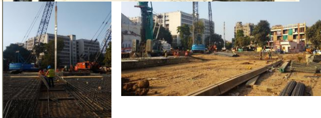
■ Metro station construction
