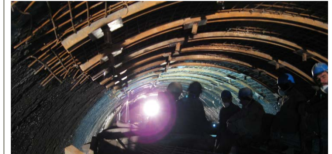
Heavy support in areas of fault zones
