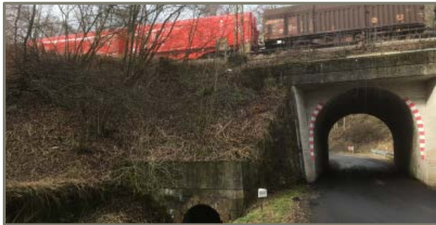
■ Culvert and railway overpass
