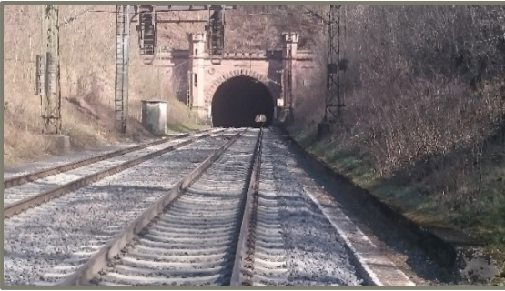
■ West portal of the existing tunnel
