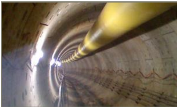
■ View of tunnel after completion of structural works
