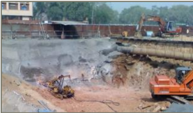
■ View of construction site
