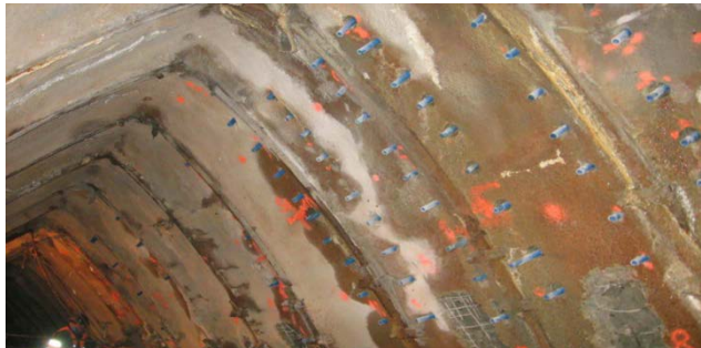
■ Injections in the core bench area
