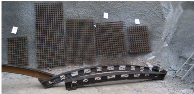
■ Specially developed steel arches for reinforcement
