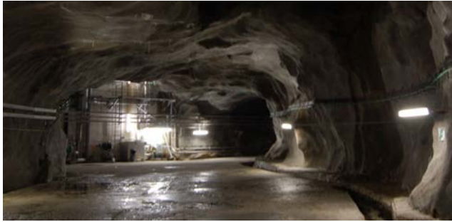
■ Access tunnel power house
