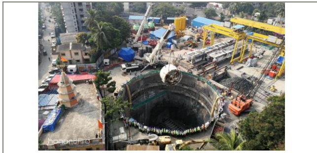
■ Aerial photo of Launching shaft construction site
