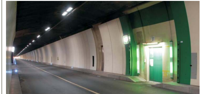
■ Tunnel after completion of renewal
