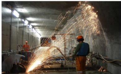
■ Step 3: Cutting of slabs in transportable pieces
