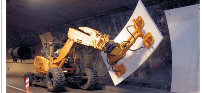
■ Step 7: Installation of wall framework
