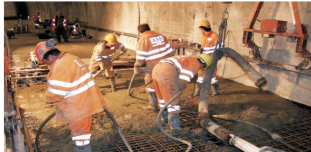
■ Step 6: Concrete casting of new roadway
