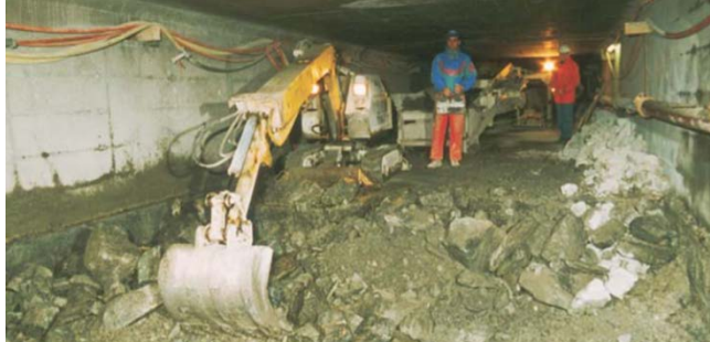
■ Step 1: Lowering of tunnel floor
