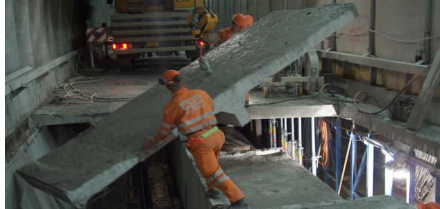
■ Step 4: Removal of cut slabs
