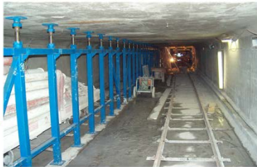
■ Step 2: Supporting of slabs in centre of roadway
