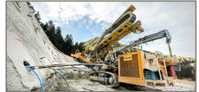
■ Reinforcement works in portal area
