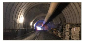
View in the direction of the east portal, transition area from the rear area to the "resumption of excavation" area with in-situ concrete acting as a means of excavation support.
