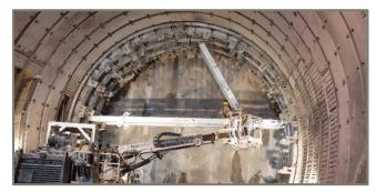
Bracing formwork of load-bearing excavation support
