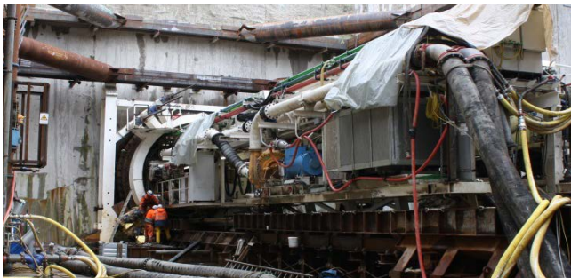
■ Installation of shield TBM
