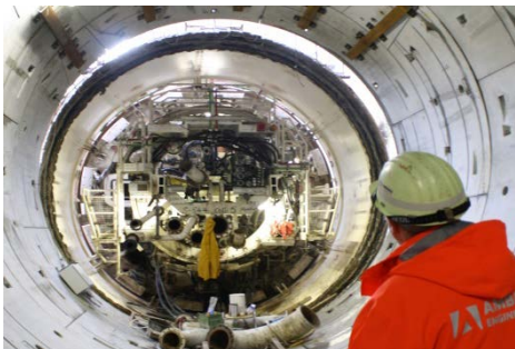
■ Shield area of TBM
