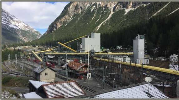
■ Site installation Preda
