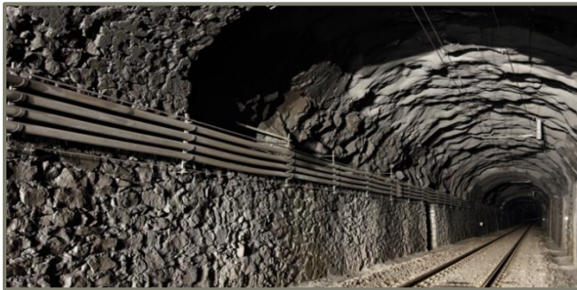
■ Old tunnel, after passing soft ground area
