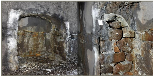
■ Old tunnel, deteriorated sections and brick lining
