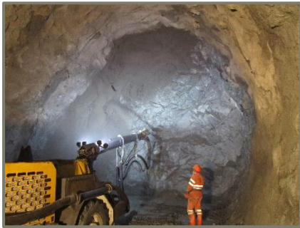
■ Drill-and-blast advance Preda
