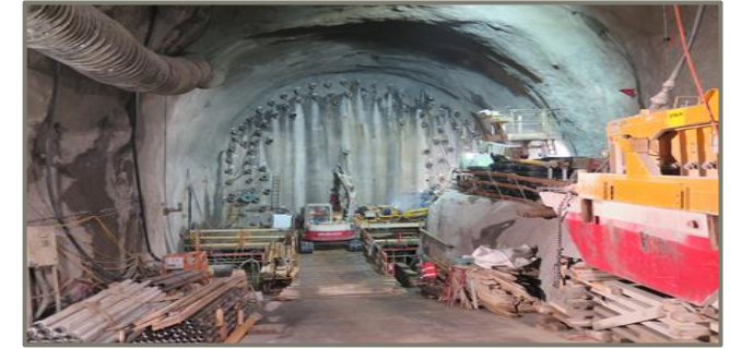
Freezing tubes at cavern at Tm 1'300
