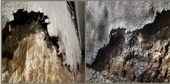
Damaged vaulted area of old tunnels
