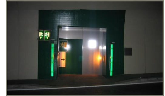
Escape door (sliding door) to the secure area
