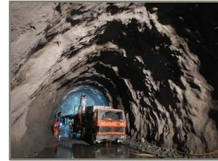
■ Drill-and-blast advance Spinass
