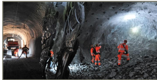
■ Merge between the old and the new tunnel
