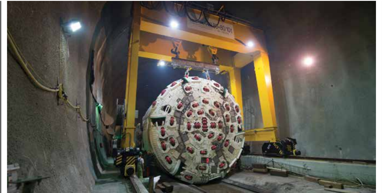
Above: Open gripper TBM for the exploratory tunnel in Ahrental
