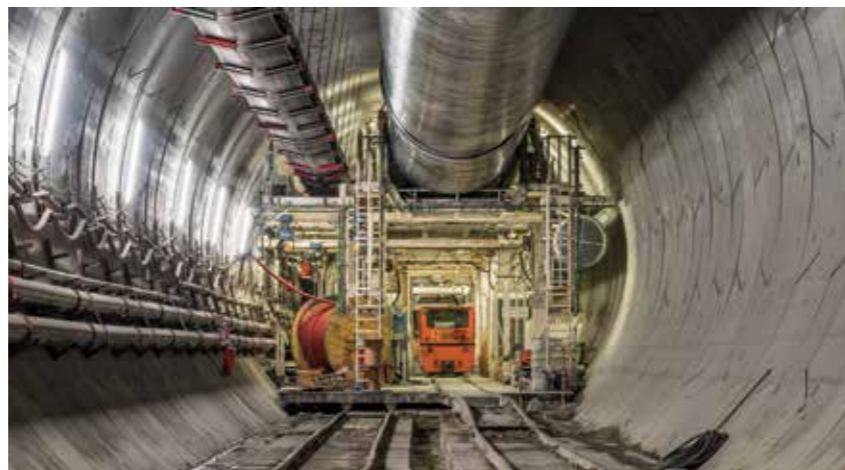
Above: TBM Flavia working on the Brenner Base Tunnel
