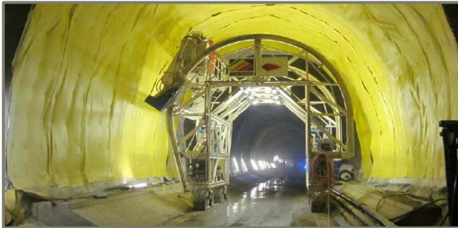
■ Sealing and establishment of lining
