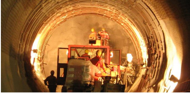
■ Rock reinforcement, fault zone using steel arches
