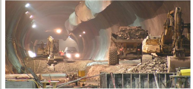
■ Mucking in the area of the south portal
