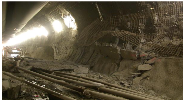
■ Rock burst at the multifunction station Faido
