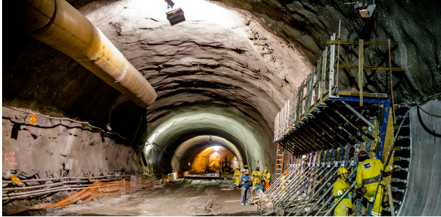
■ Excavation of Rio450 tunnel
