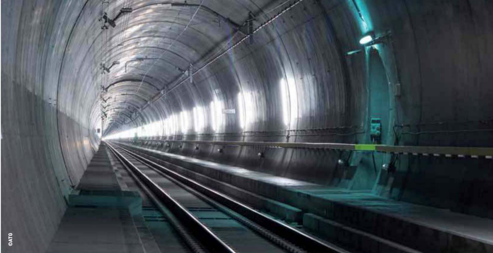
→ The Gotthard Base Tunnel after installation of the rails and railway equipment.
