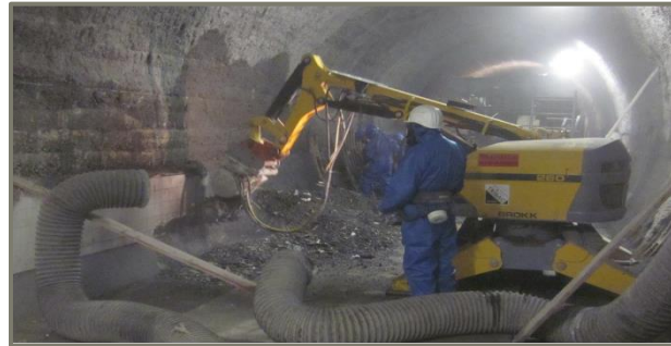
■ Removal of lining concrete
