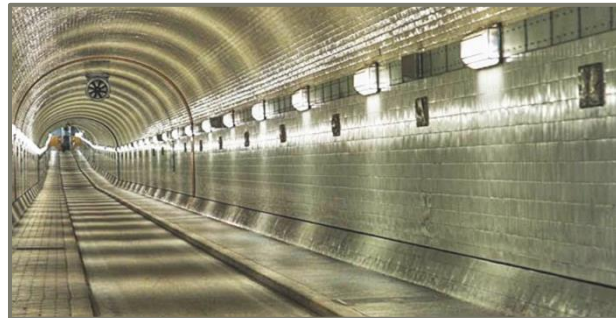
■ After restoration, showing new installations (safety)
