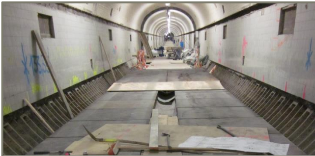
■ New sealing and utility ducts in roadway area
