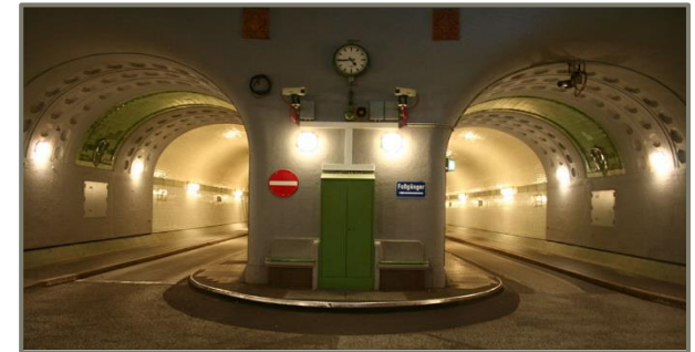
■ View of subsurface tunnel portals
