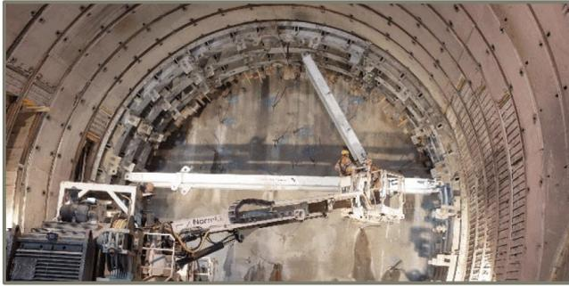
Bracing formwork of load-bearing excavation support
